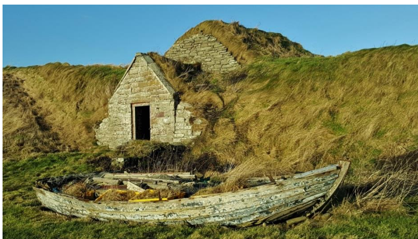
Figure 9. The abandoned ice-house and salmon coble at Keiss fishing station in Caithness. The packing station is at the front of the ice-house. The ice-store is to the rear and was charged from the upper level via a hatchway let into the turf roof.
